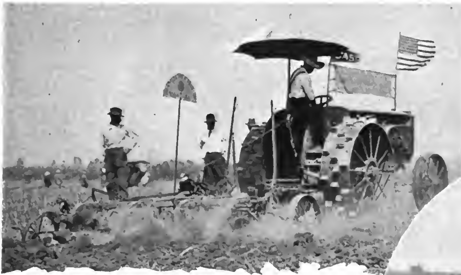
Below—The "Happy Farmer," a tractor in which the weight is very little forward of the driving axle
